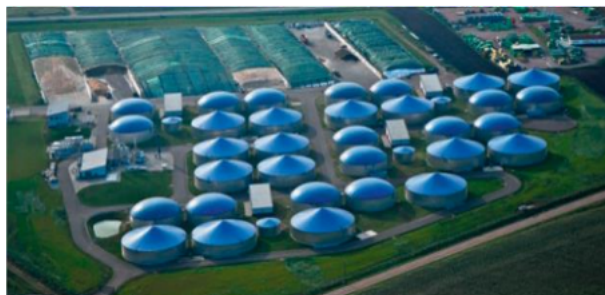
Fermentory a sklady digestátu na bioplynové stanici Digester, secondary digester and end storage of digestate of a biogas plant
